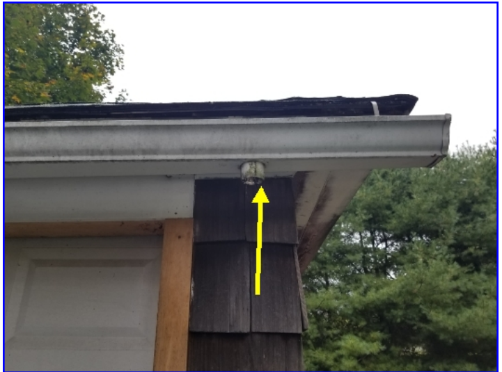
Gutters to garage were disconnected and not functioning. The inspector recommends having licensed contractor replace.
