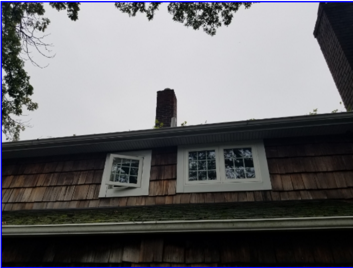
Debris visible in the gutters at the time of the inspection should be removed to encourage proper drainage.
