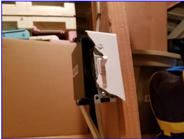
Light switch broken cover.
