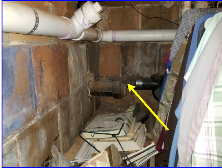
Main clean outs located in basement.
