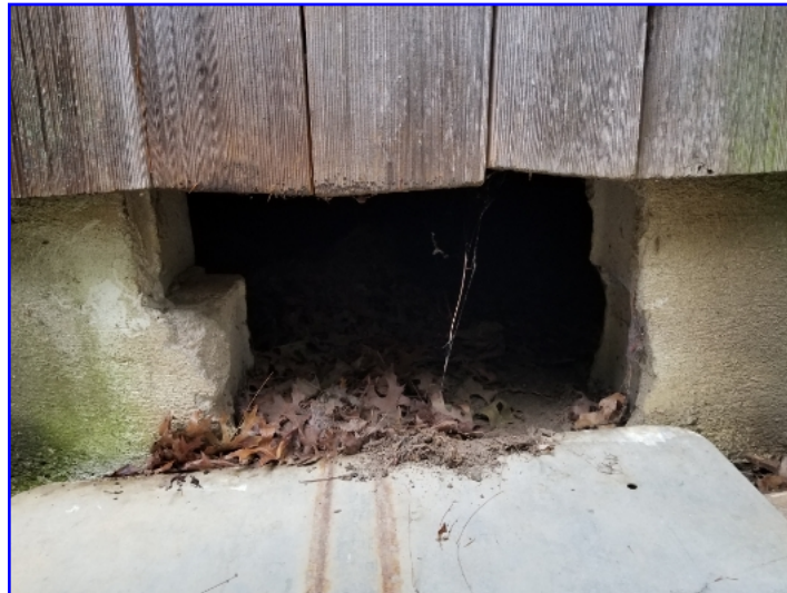
Crawl space window was missing window at time of inspection. The inspector recommends installation by licensed contractor.
