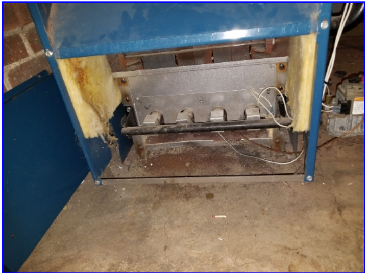
The boiler was dirty. The Inspector recommends having boiler cleaned by a qualified HVAC technician.
