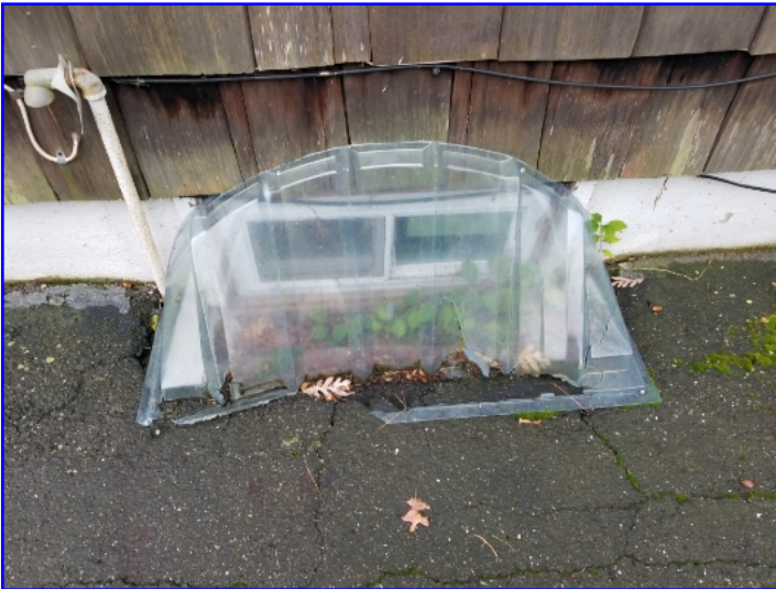
A window well was not securely attached to the home structure.
