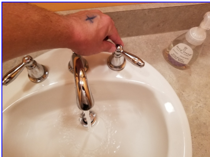
The bathroom sink faucet was loose and should be mounted more securely.
