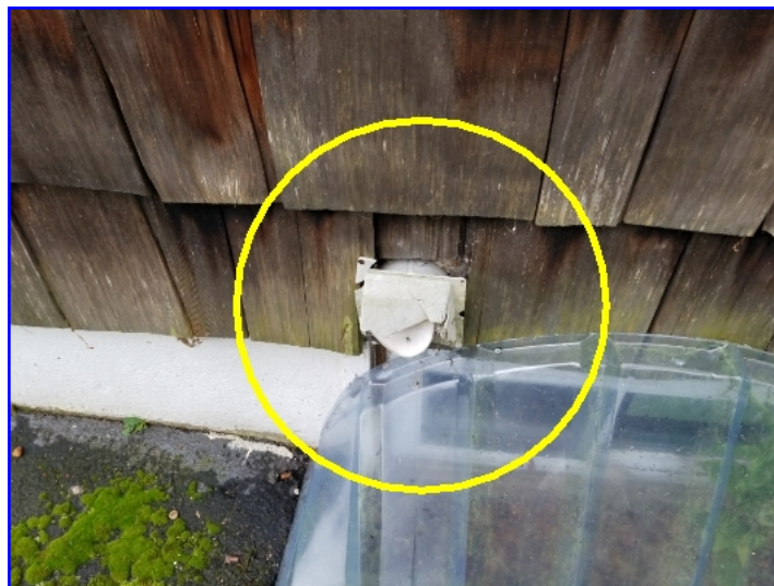
Dryer vent cover is damaged.
