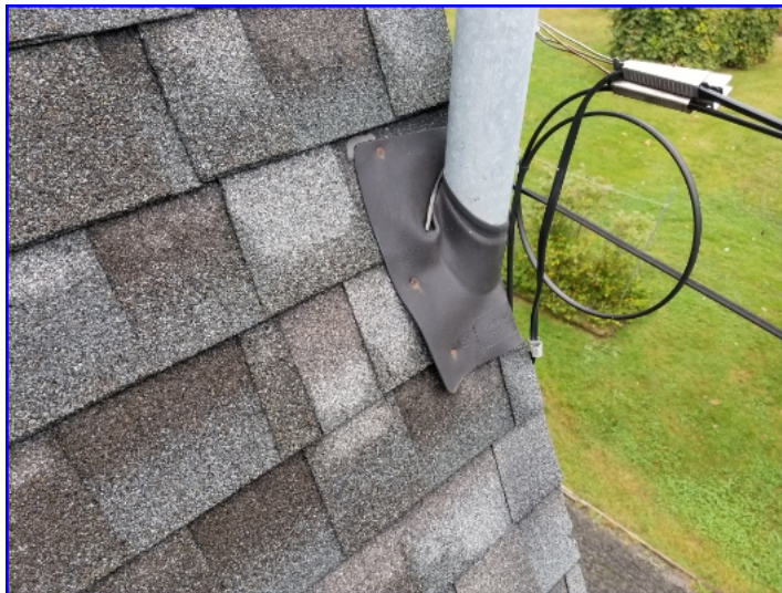
The point at which the electrical mast penetrated the roof-covering material did not have proper flashing installed. The inspector recommends correction by a qualified roofing contractor.
