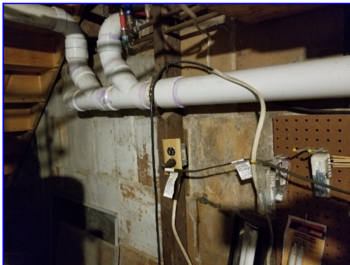
The visible drain, waste and vent (DWV) pipes were a combination of cast iron and approved PVC.
