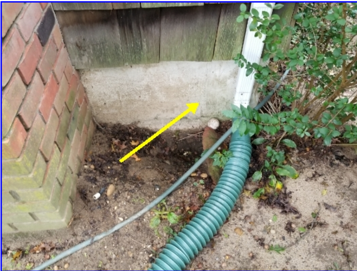
All cracks in exterior block and parge coat should be filled and sealed.
