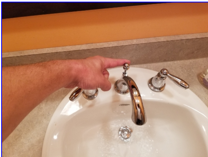
The sink in this bathroom had an inoperable stopper.
