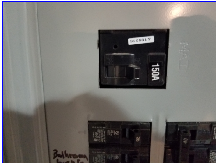
The electrical service disconnect was rated at 150 amps.
