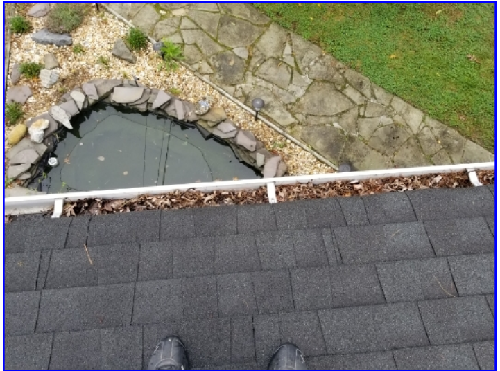
Debris visible in the gutters at the time of the inspection should be removed to encourage proper drainage.
