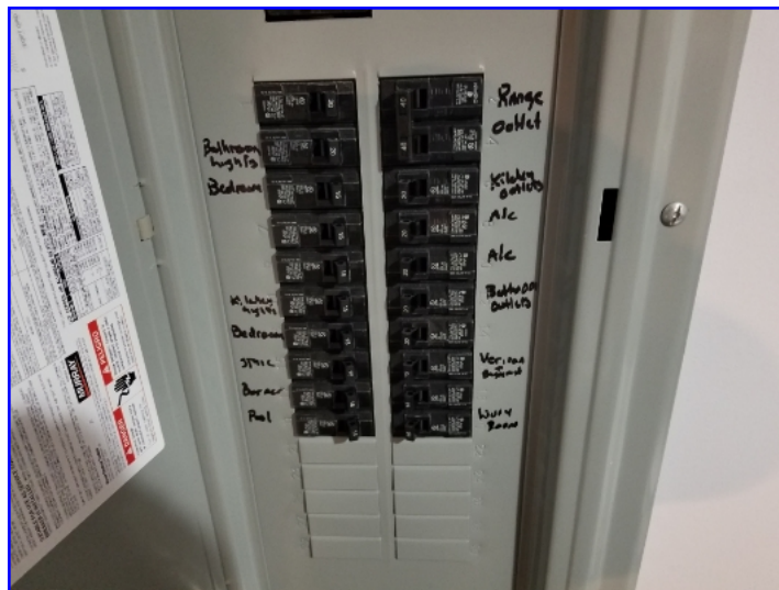
The Circuit Directory label for the service panel is shown in the photo.
